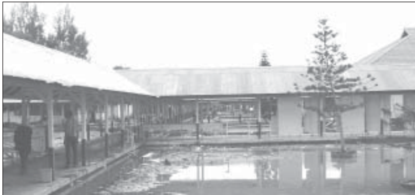
Banda Aceh Hospital, still wet weeks after the tsunami
